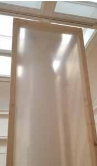
Columns under plastic
